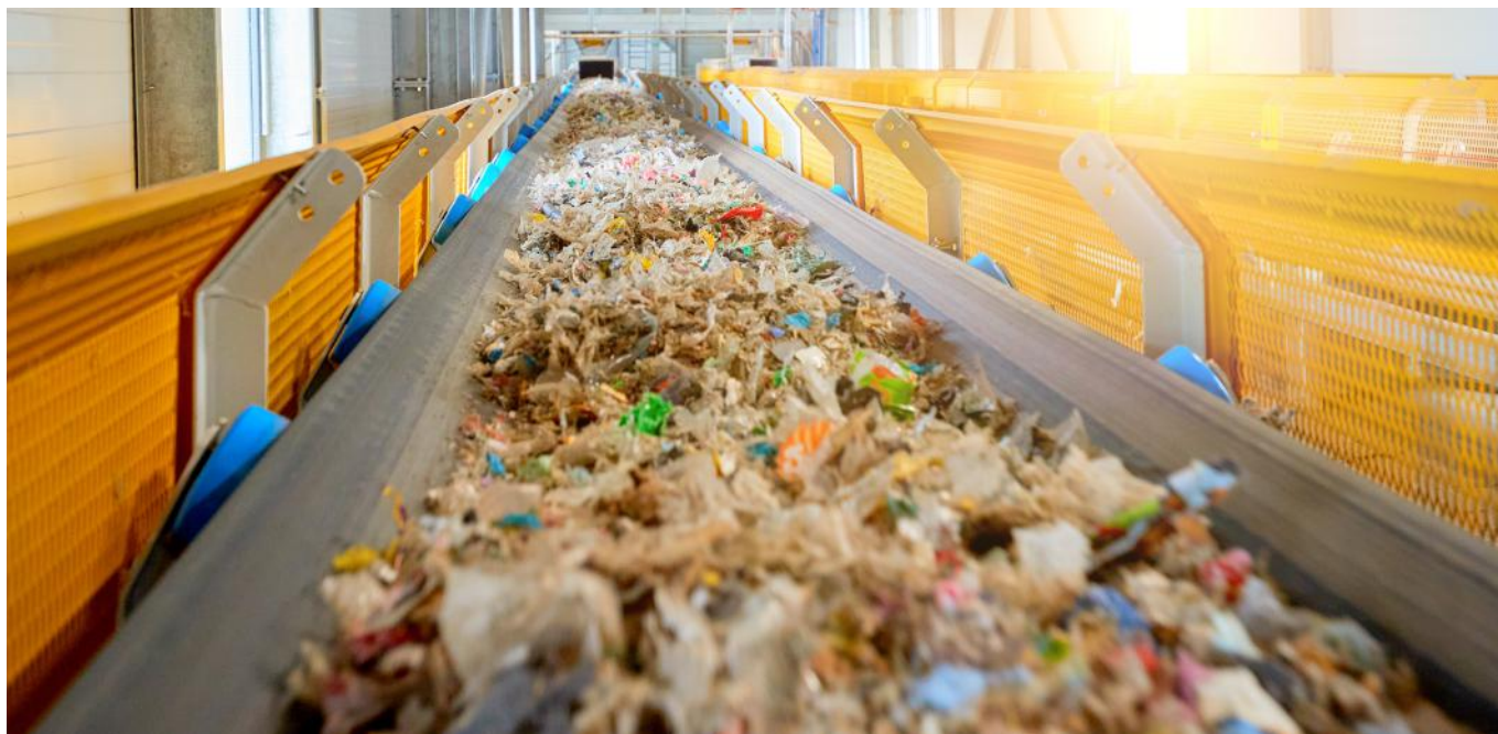
Fuel conveyor: municipal solid waste on its way to a boiler for combustion. Photograph: Martin Mecnarowski via Shutterstock
