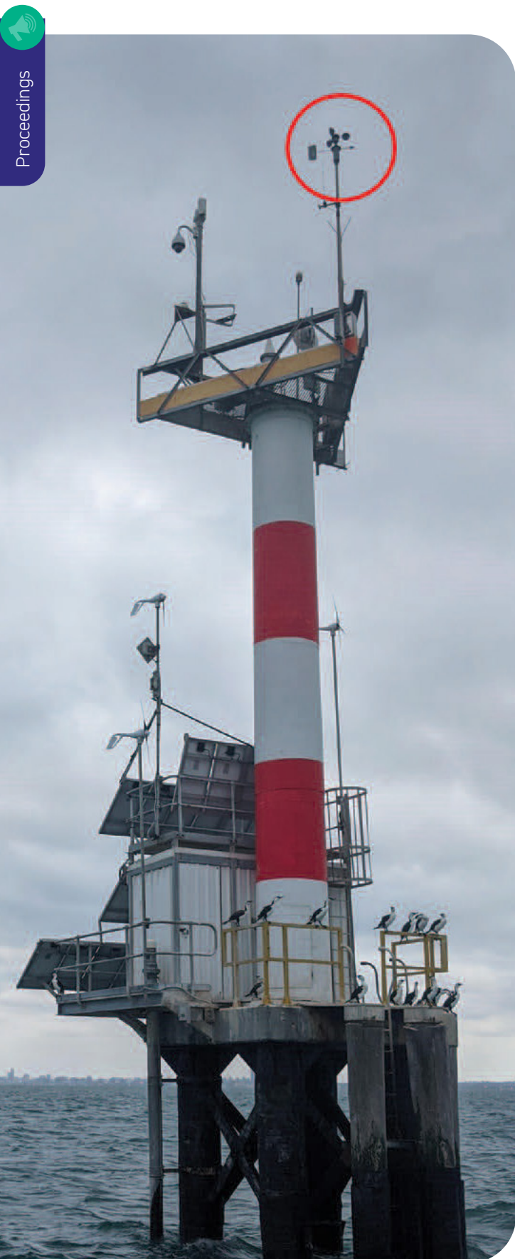
The Fawkner Beacon (the anemometer with direction vane is at the highest point on the tower — shown ringed in red).
