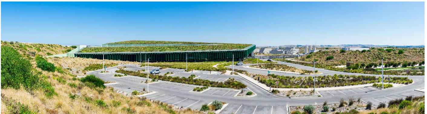
The Victorian Desalination Plant at Wonthaggi was completed in 2012. It can produce 410 megalitres of water per day.
