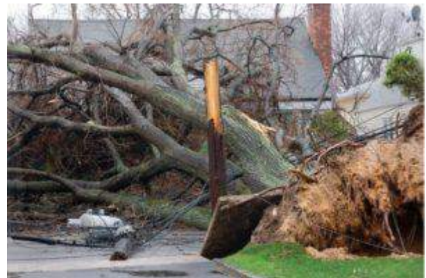
Uprooted tree damaging electricity network equipment (Credit: Nycshooter/E+/Getty Images).
